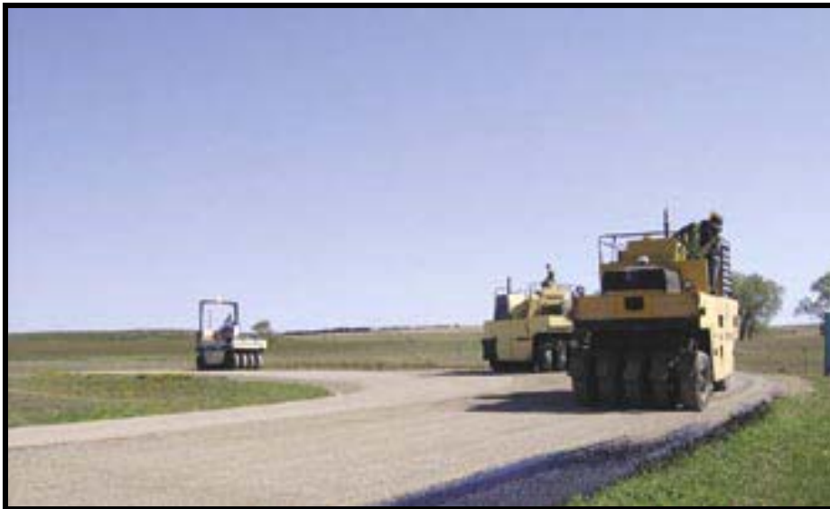
Rollers finishing the newly chip sealed road.
