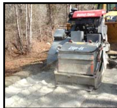
Elmore County uses an Asphalt Zipper reclaiming-milling attachment that works with a loader.
