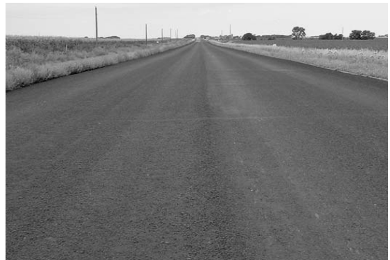
A fog sealed chip seal virtually eliminates windshield damage to vehicles.
