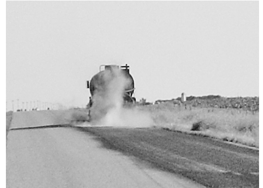
Fog seal being applied in Hutchinson County.
