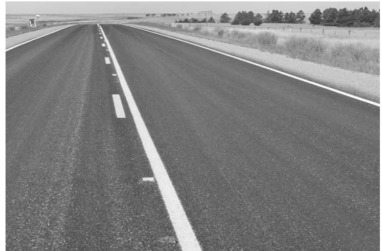
Pavement markings show up very clearly after fog sealing.
