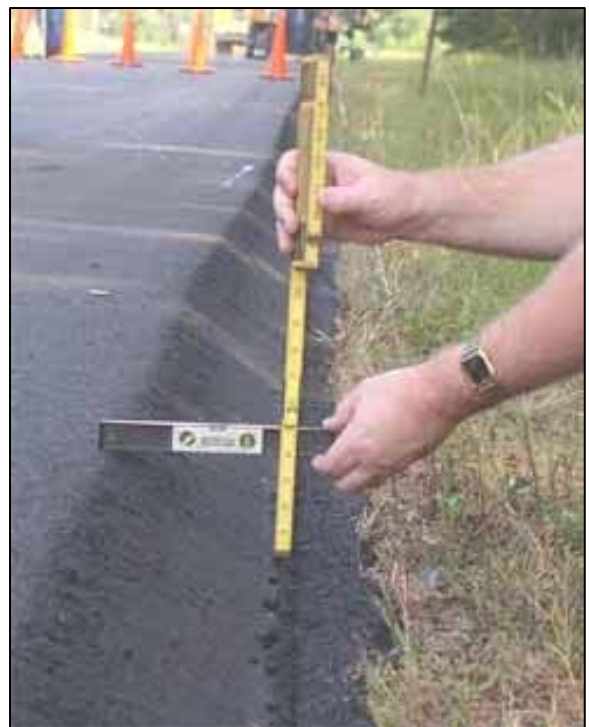
An inexpensive way to assure safe pavement edges is to specify a 30 degree to 35 degree angle asphalt fillet "Safety Edge" on all road construction and resurfacing.
