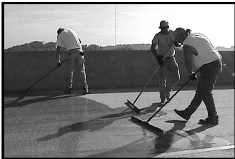
The first coat of polymer is applied with a notched squeegee.
