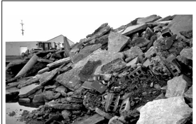
Mitchell stockpiles both salvage asphalt and concrete and then crushes and blends both materials for use as base in new construction.
