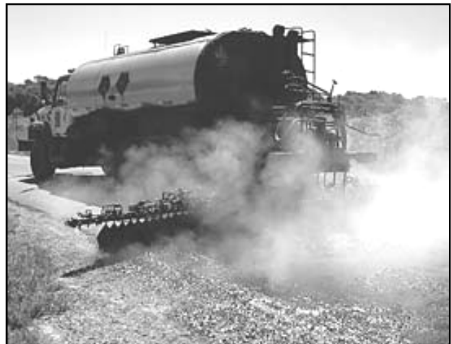
Work on a chip seal project.
