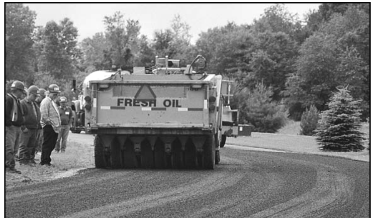
Rubber tire roller imbedding aggregate on a chip seal project.
