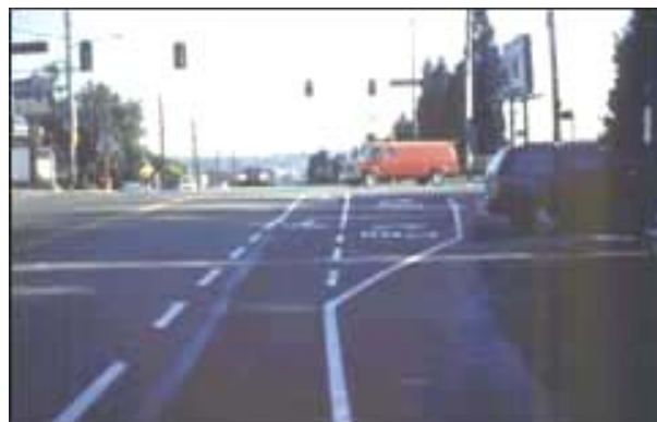
Approaching major intersections with right-only turns often calls for additional striping close to the intersection. "
