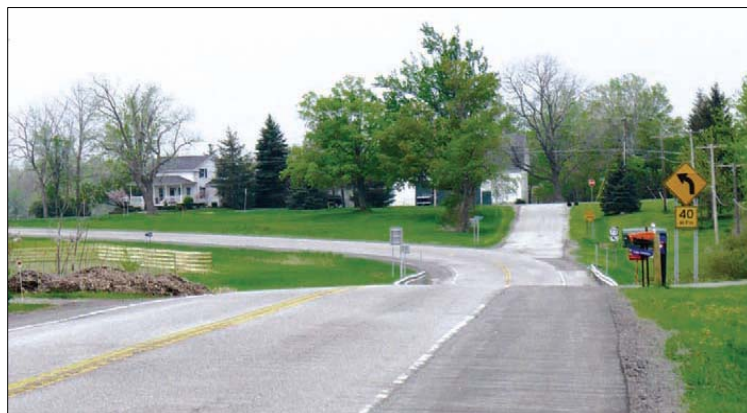
Figure 1: Major road turning to the left with a minor road going straight
